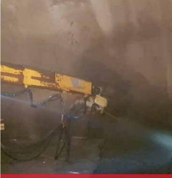
Tested in controlled site facilities , the amount of rebound is calculated according to the weight of rebound. Using 18.5% of CEM II rebound may be controlled to just under 8.5%
